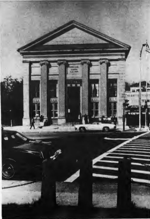
QUINCY CITY HALL, erected in 1844, is a handsomely designed granite and pillared building, located in the heart of Quincy Sq.
